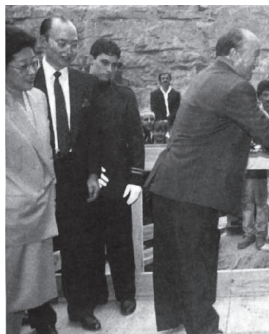
Father throws the first shovelful of dirt onto the initial construction work for the new tower.
